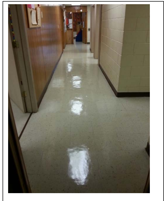
The new finish on the Learning Center on 12 th Street.
