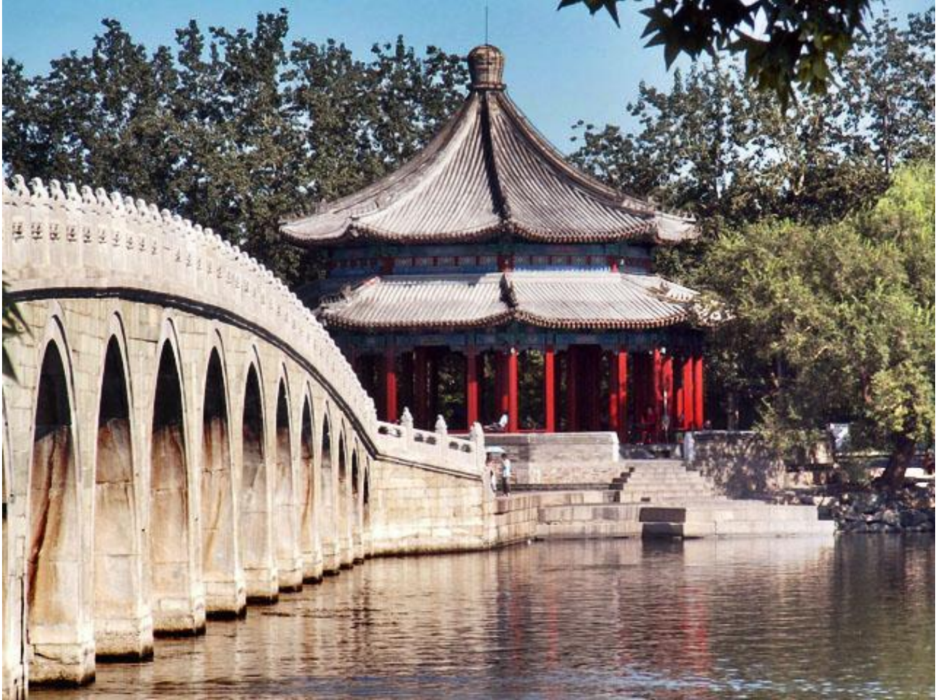
The Seventeen Arch Bridge – Summer Palace
